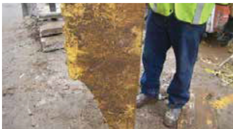
Roadway Insulation Minneapolis, MN
