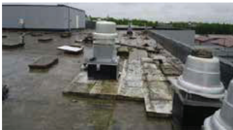
Roof B Wasilla, AK
