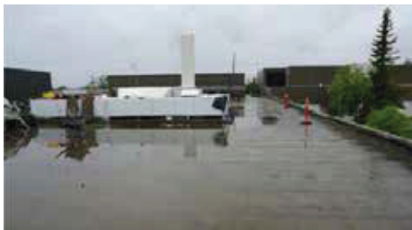
Roof A Wasilla, AK
