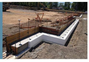
The Expanded Polystyrene Association of Canada (EPAC) conducted a joint research project with the National Research Council of Canada/Institute for Research in Construction (NRC/IRC) to evaluate the durability performance of expanded polystyrene (EPS) insulation in an exterior below-grade application. EPS insulation, thermal performance, site weather conditions and soil moisture content were instrumented and monitored throughout the project.
